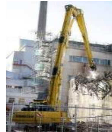
Decommissioning and environmental remediation
