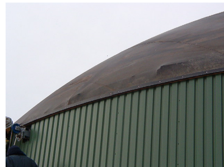
Damages at the wooden beam construction in fermenter
